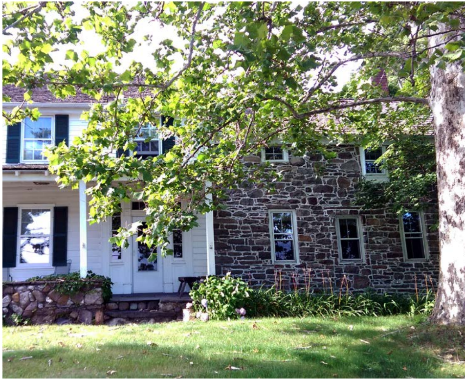
Greycourt Manor, William Bull's first stone building project in America, was razed in 1832. This smaller companion stone building was probably completed next. The Roe family added the large frame extension around 1840.
